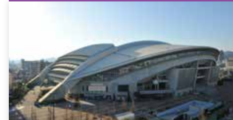
Kobe Misaki Stadium
