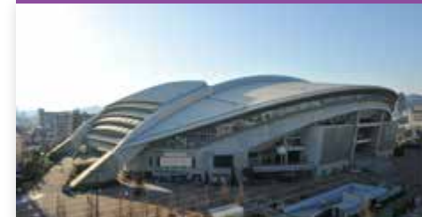
Kobe Misaki Stadium
