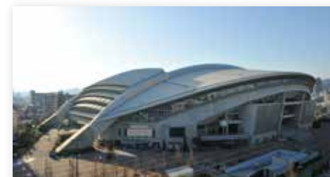
Kobe Misaki Stadium
